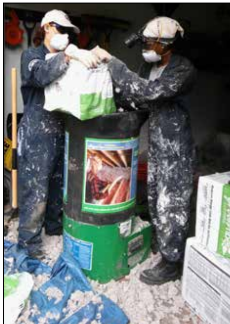
National Civilian Community Corps members Jenna Uretsky(left) and Keziah Little pour cellulose into the hopper to prepare it for use as attic insulation.
